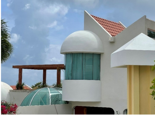
Concrete and glass volumes
