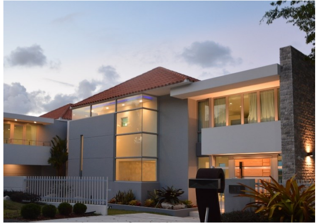
Concrete and glass volumes
